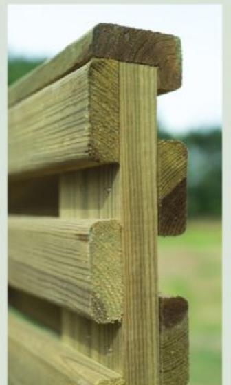
Discreet fixings create a genuine dual faced panel. For a seamless run the panels can be supported from the back.
